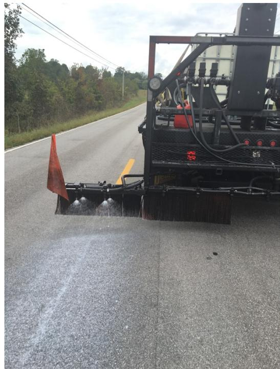
THE PAVEMENT RESTORATIONS CREW AND EQUIPMENT APPLYING BIORESTOR TO CELENA HIGHWAY NEAR ALLONS IN NORTH CENTRAL TENNESSEE. (PHOTO CREDIT: JON HARGETT)
