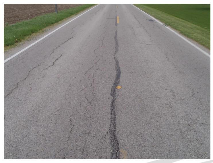
Image clearly shows accelerated weathering, further defined and development of longitudinal cracking and alligator cracking
