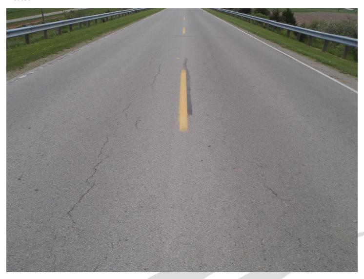
Image clearly shows lighter weathering, longitudinal cracking and alligator cracking
