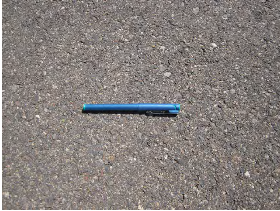
Figure 3: Typical asphalt surface suited to enrichment.
