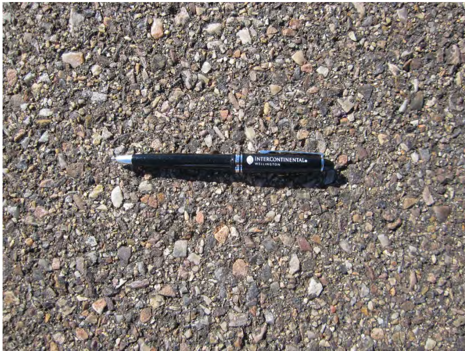
Figure 4: Typical asphalt surface suited to surface filler.
