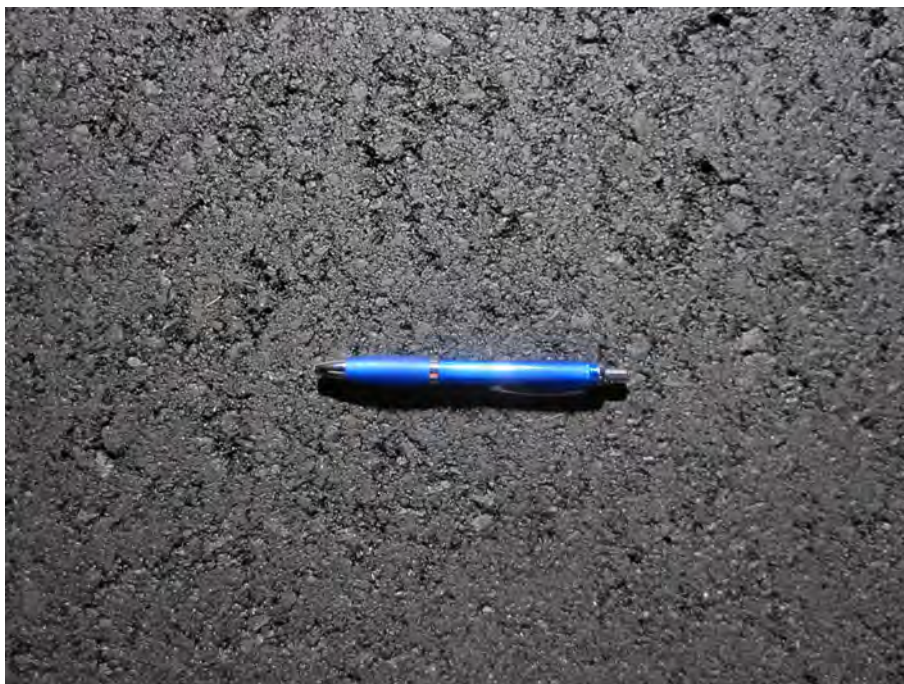
Figure 2: Typical asphalt surface suited to rejuvenation.
